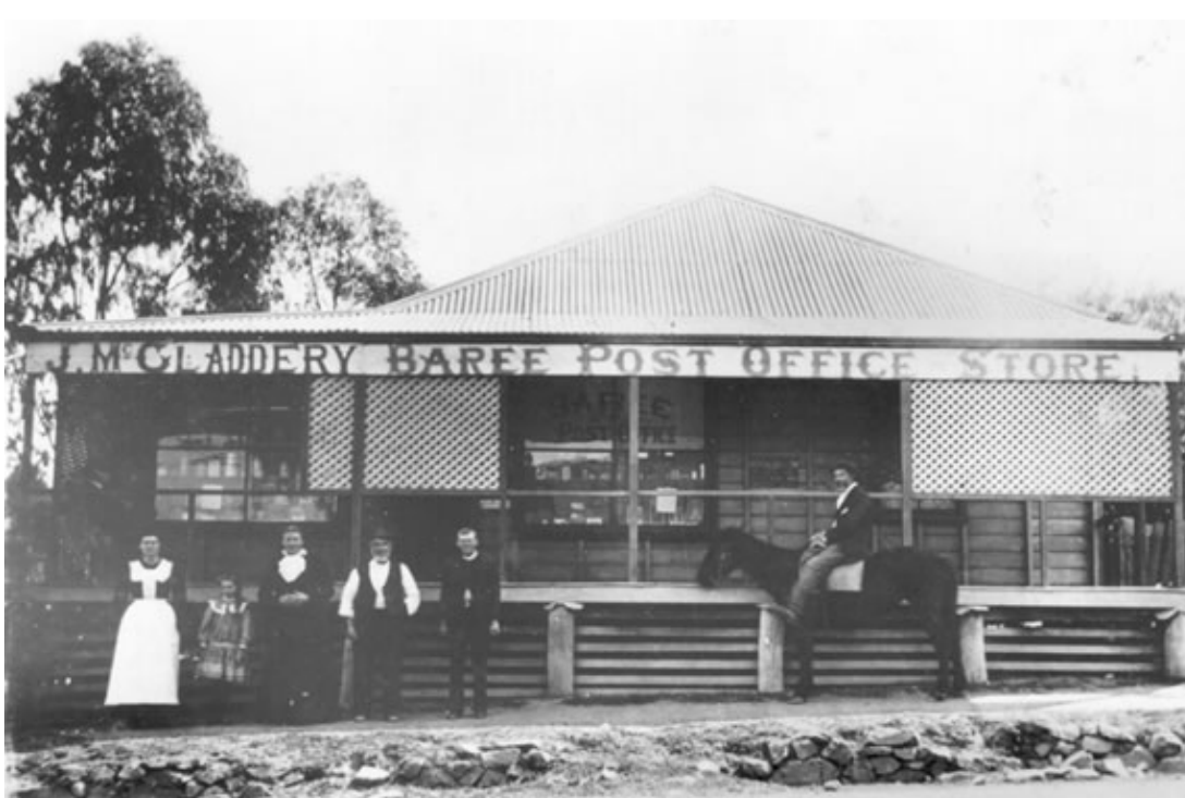
Fig. 11. Baree Post office and store, c. 1918. Wide horizontal cladding to interior, exposed external timbers, enclosed verandah on left with skillion roof provides shop space. Frontage to the road is terraced to the ground level of steps, right, near split slab fence. Wide metal plates above foundation posts of bush timber protect against white ants.
