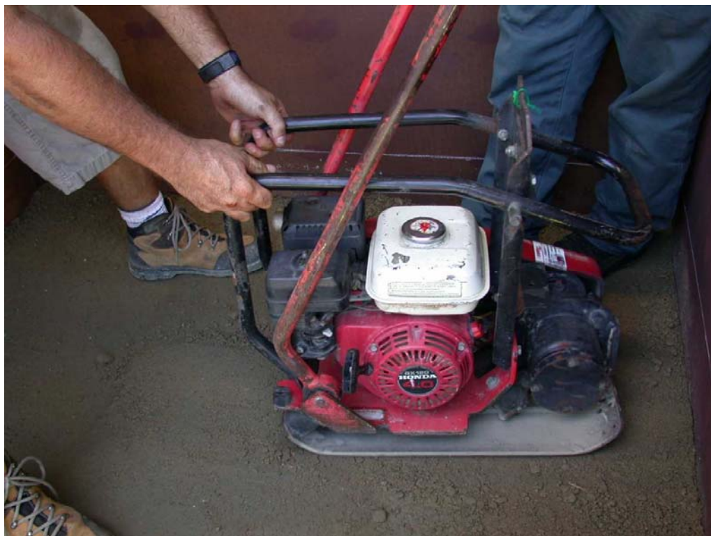
Figure 6.15 Compaction using a 40kg plate compactor
