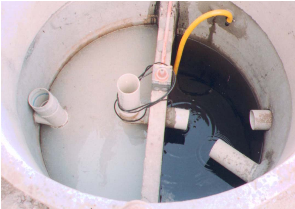
Figure 2.11 Interior of Rockhampton Holding Tank
