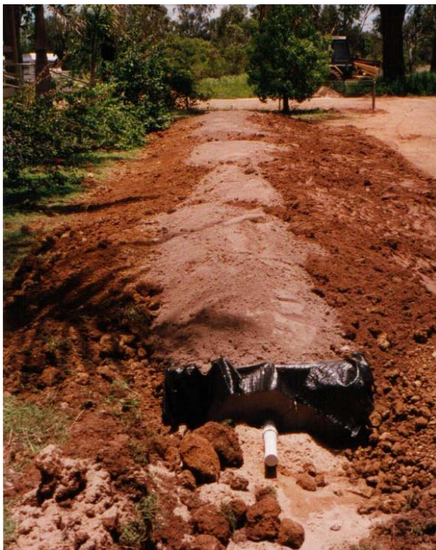
Figure 2.9 Soil filled RET channel at Anakie site
