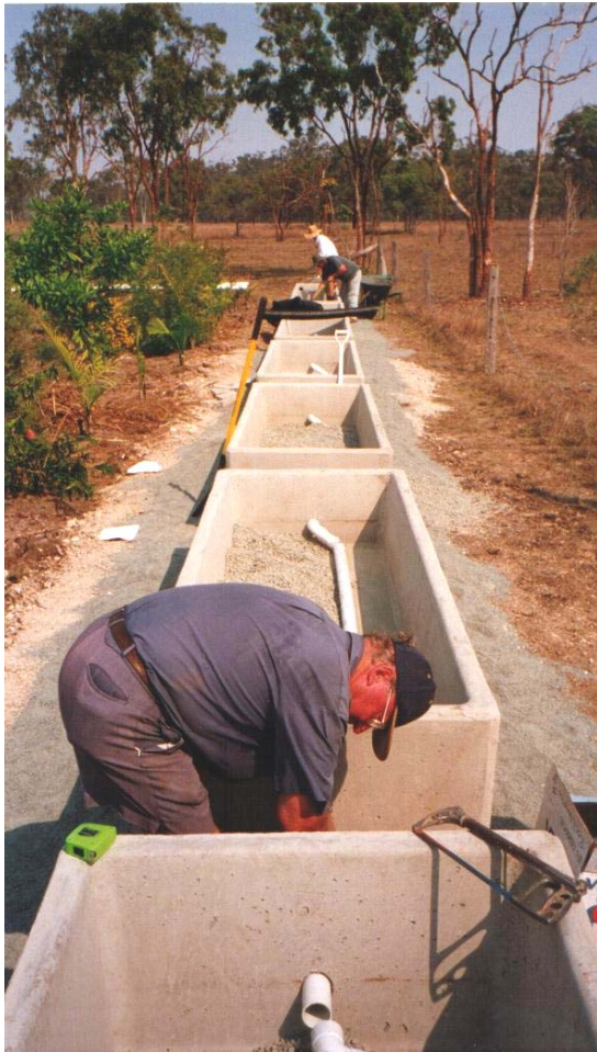
Figure 2.8 Pipework and aggregate in RET channel-to-channel flow-through design
