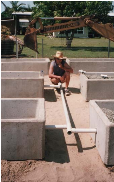
Figure 2.7 Herringbone RET channel design with central feed line
