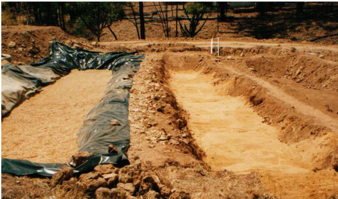
Figure 2.13 RET channels at various stages of construction at Gem-Air caravan park
