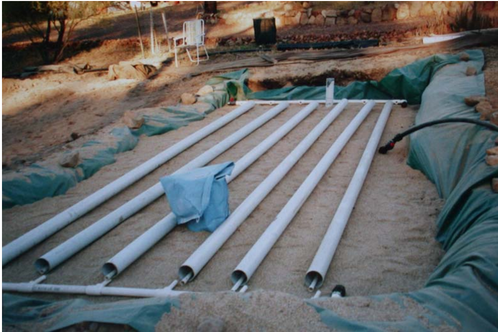
Figure 2.14 Recirculating sand-filter showing effluent distribution system
