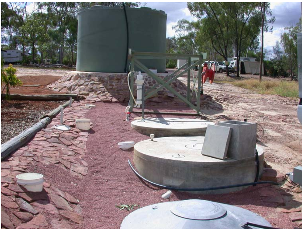
Figure 2.15 Gem-Air treatment tanks
