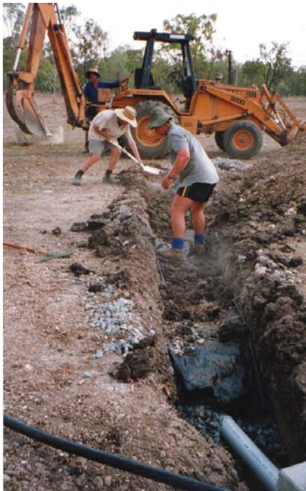
Figure 2.5 Construction of emergency overflow at Yaamba trial
