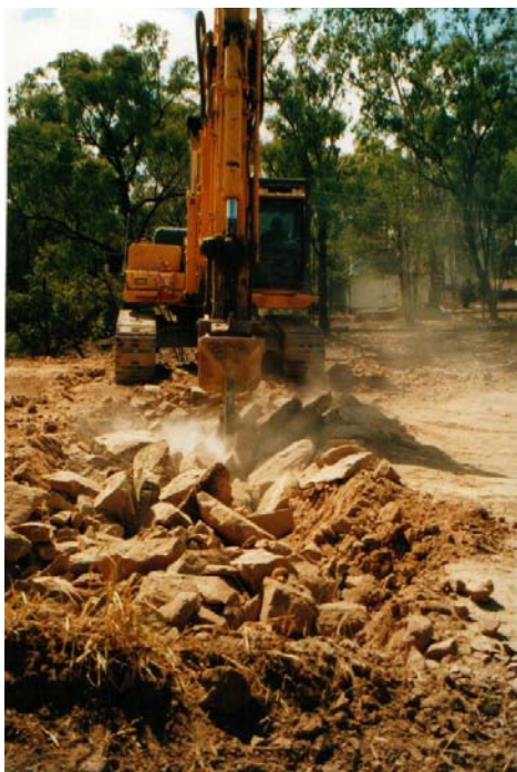
Figure 2.12 Digging RET channels in sandstone at Gem-Air caravan park
