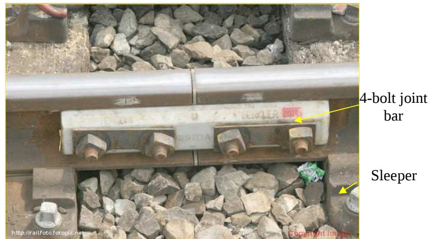
Figure 2.1 Suspended IRJ (RAILFOTO, 2005)
