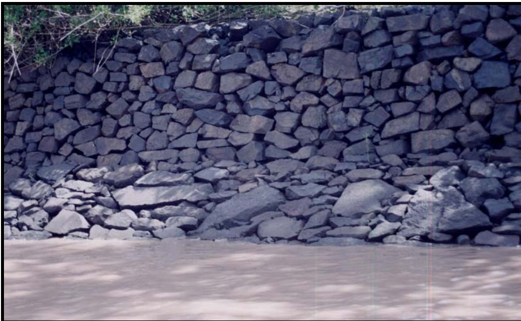
Close-up view of The Stone Wall dry-stone paving.
