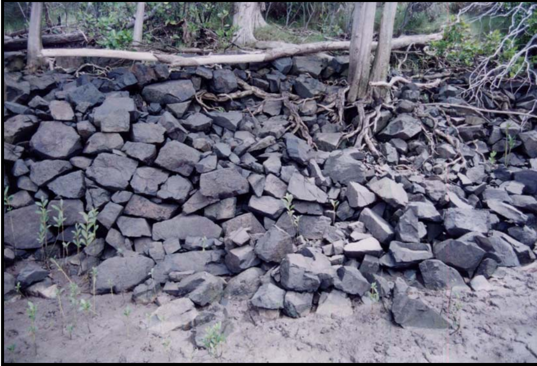
Tree roots breaking stonework.
