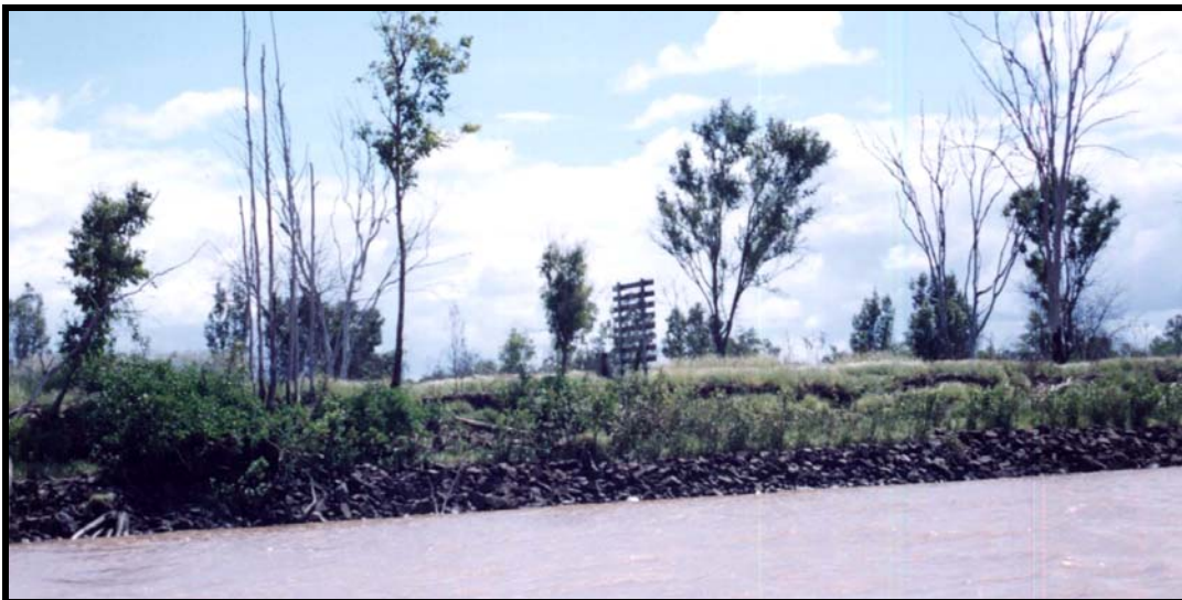
Start of stone walls on south bank, No. 1 wall, now decayed, with lead board to direct pleasure boats up the river.
